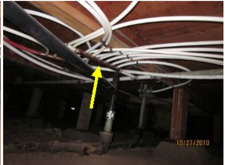
Manifold for Pex piping
