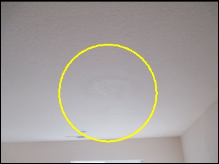
Visible repairs at loft ceiling
