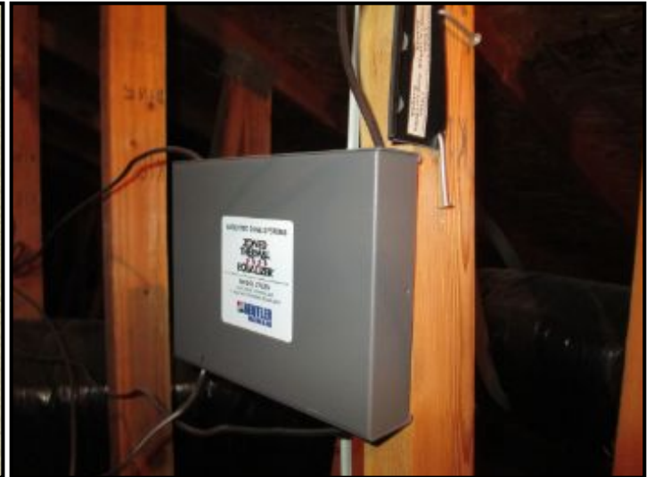
Dual zone control in attic
