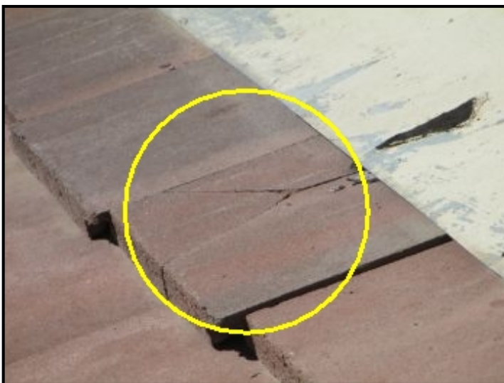
Damaged tile front of house
