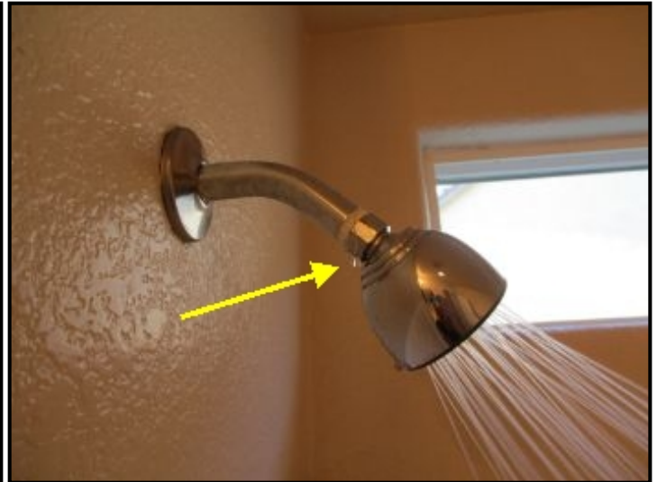
Shower head leaks at connection, Bath 3
