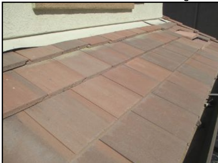
Damaged tile front of house
