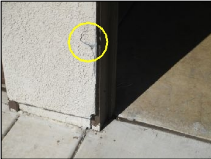
Minor stucco damage
