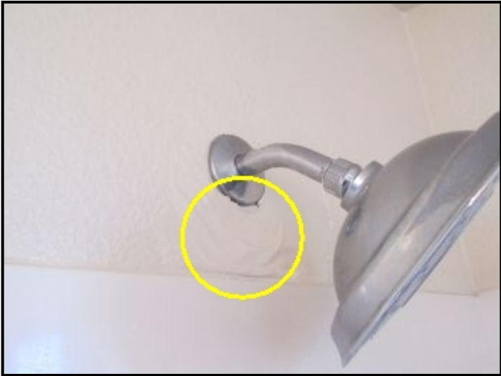
Paint peeling under shower head, M bath
